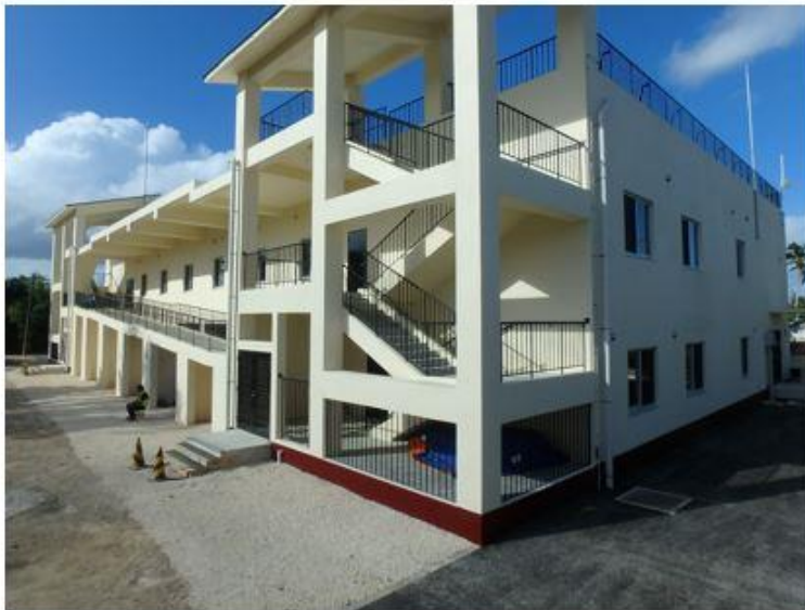
HQ & Studio Building
