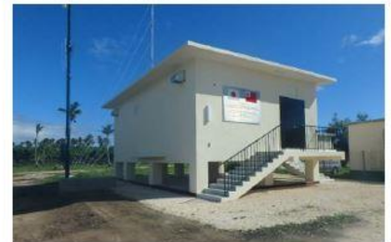
MW Transmitter Hut
