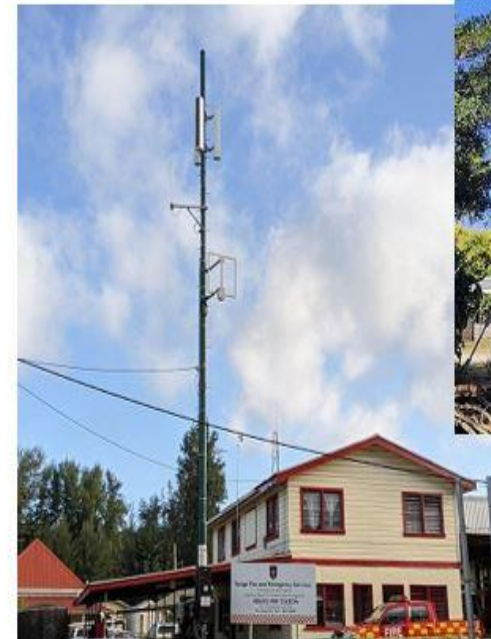
Siren Mast (RAR Control)
