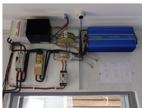
Photo-20 : Battery Controller and Inverter (2014.7.1)
